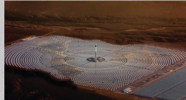
Central solar Noor Ouarzazate III, Marruecos. Fuente: Masen - Moroccan Agency for Sustainable Energy, 2025.
