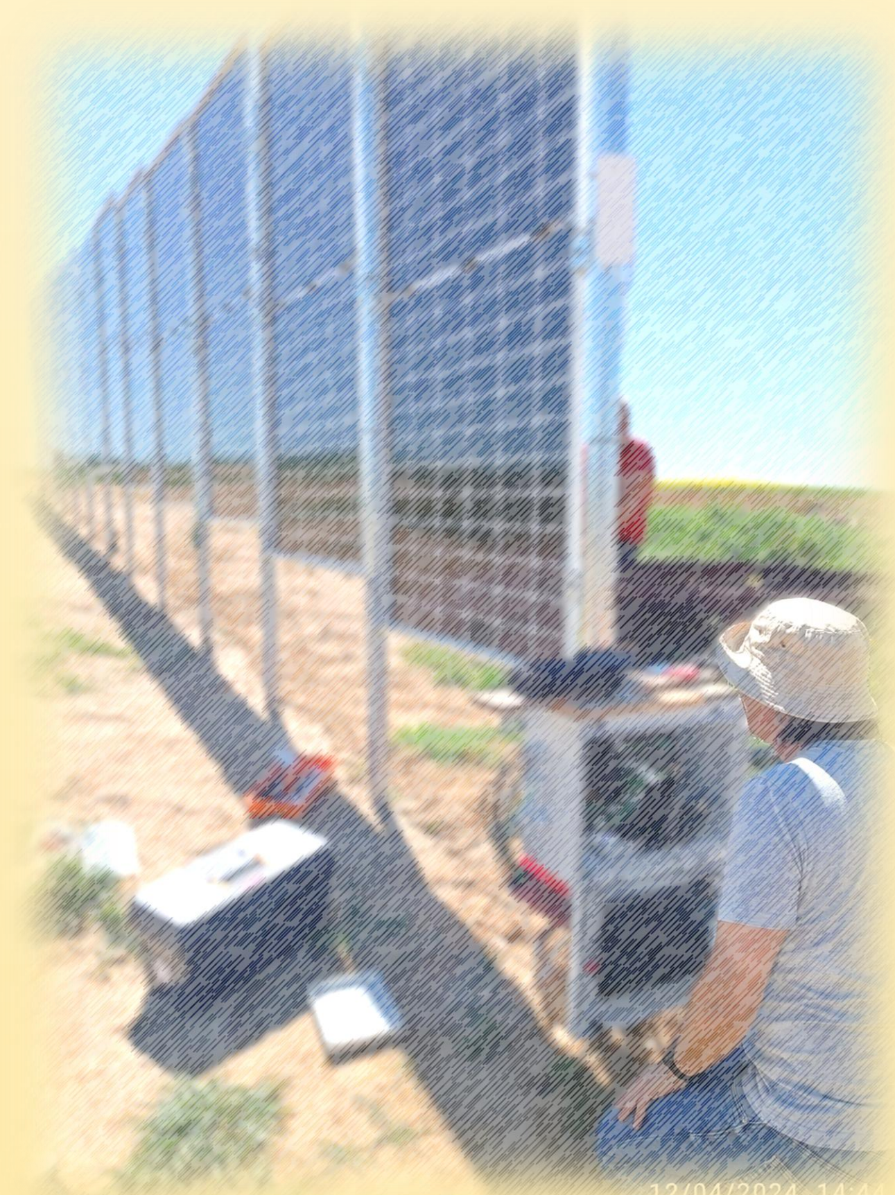
Figure 1: Agrivoltaic system with vertical bifacial PV panels.
