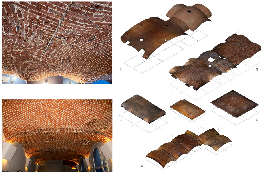
Fig. 1. Examples of low brick vaults by slices in Turin with concentric brickwork, metal tie rods and diagonal brickwork.
