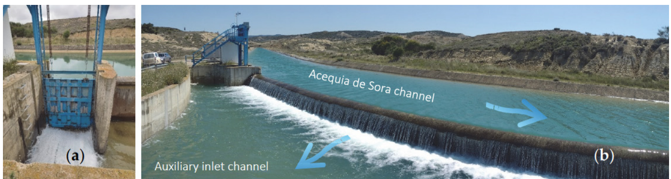
Figure 2. Intake work in the Acequia de Sora channel: (a) View from downstream of the flow control gate in operation. (b) Flow control structure on the left and side spillway from the Acequia de Sora to the auxiliary channel.
