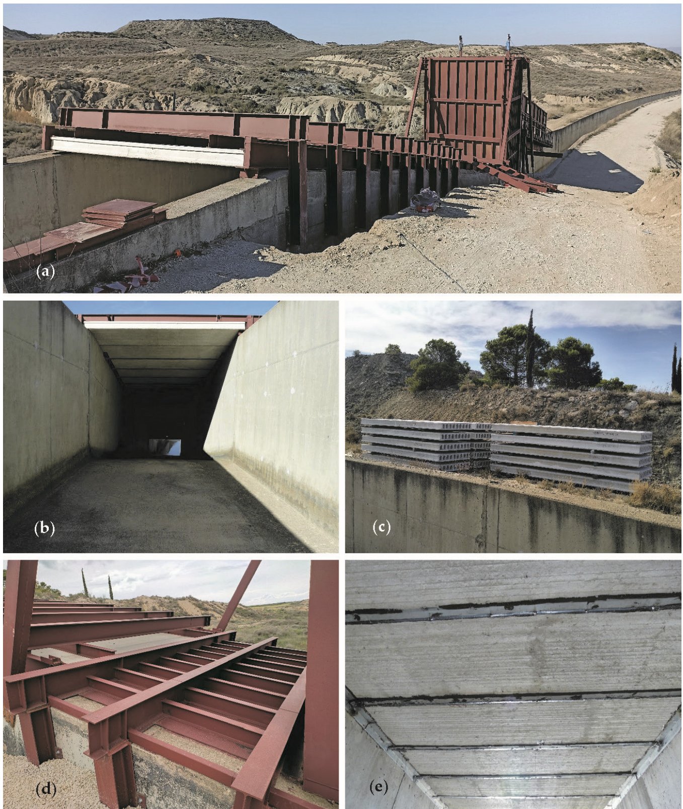
Figure 4. (a) View of HEFLR from the right bank of the auxiliary channel. (b) View of the interior of the auxiliary channel from upstream of the pressure channel. (c) Storage of the honeycomb slabs used to cover the pressure channel. (d) Metallic frames used to support the honeycomb slabs of the pressure channel and the metallic plates on the connection to the tower supply. (e) Detail of the sealing between the slabs and the channel walls (view from inside the pressure channel).
