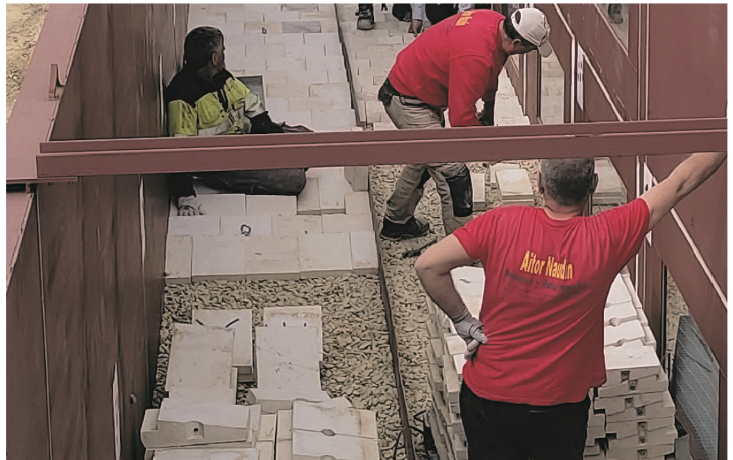
Figure 6. Picture of the placement of the WSB on the gravel bedding layer.
