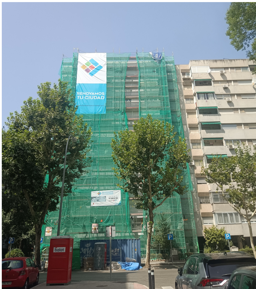
Figure 5.11: Image of a building undergoing retrofit construction in Poblado de Orcasitas
