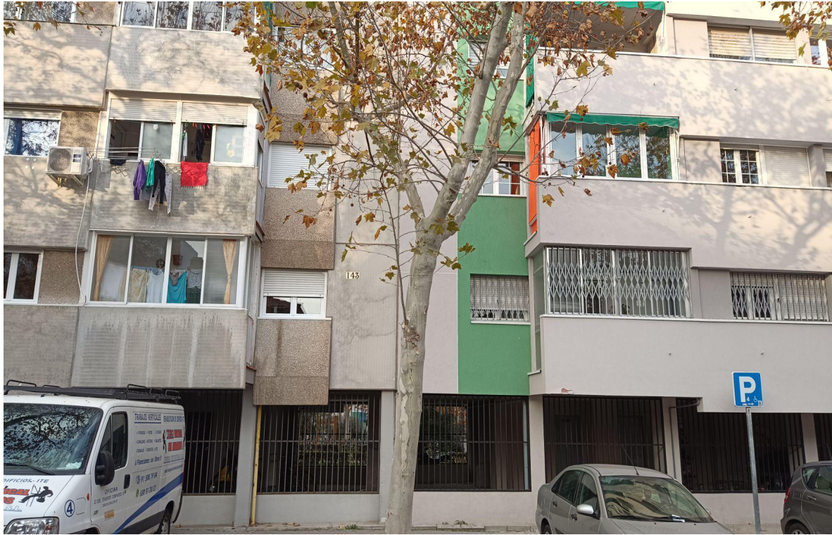
Figure 5.20: The before and after: building without retrofit on the left, and building retrofitted on the right. Poblado de Orcasitas neighbourhood
