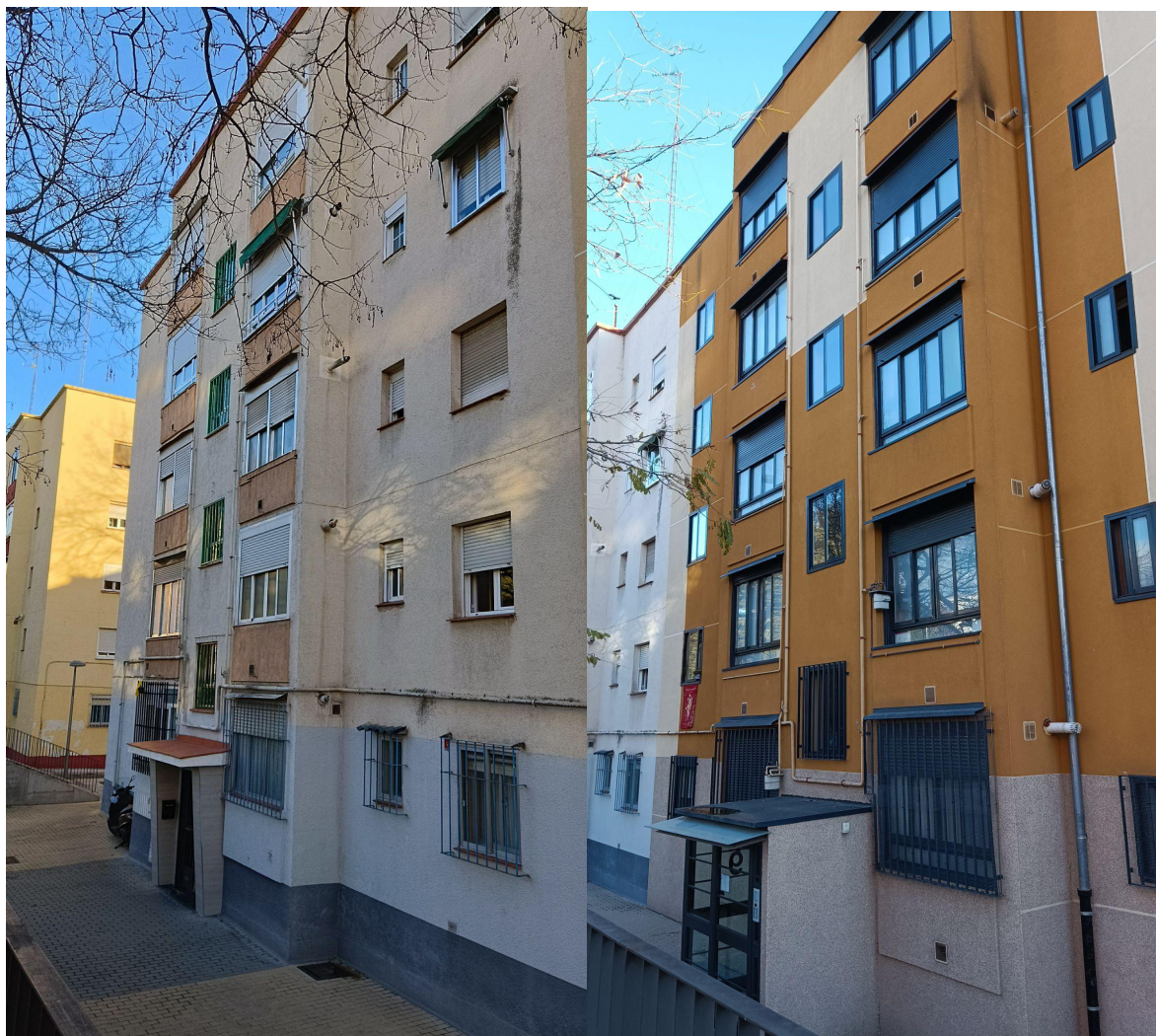
Figure 5.18: The before and after: building without retrofit on the left, and building retrofitted on the right. Ciudad los Angeles
