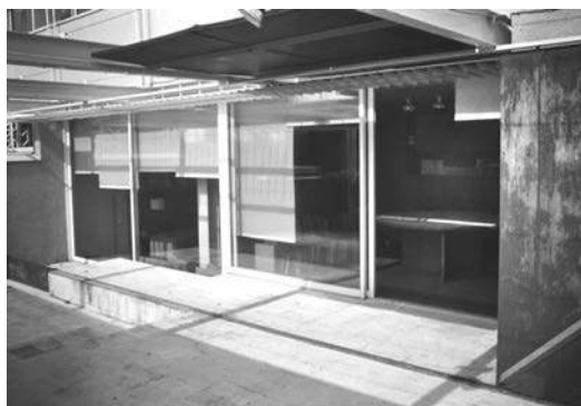
Figure 4 Porch of Corrales House. Filter and steps.
