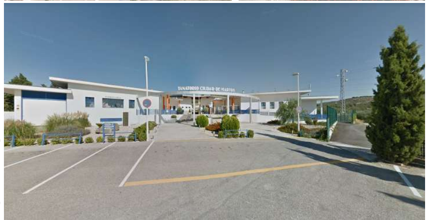
Exterior Google Street View, sept. 2019
