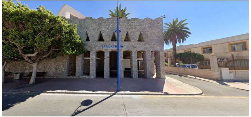
Exterior Google Street View. sept. 2022
