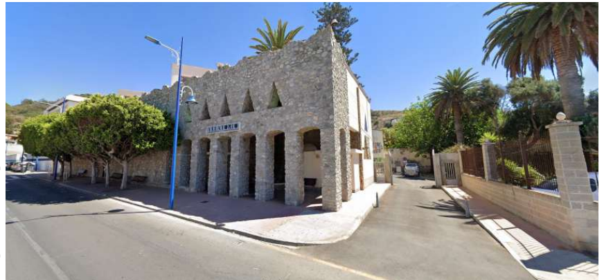
Exterior Google Street View. sept. 2022
