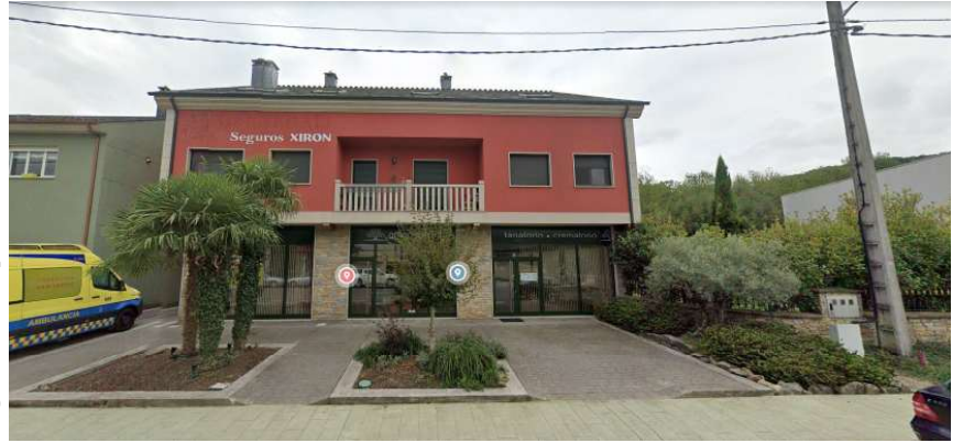
Exterior Google Street View: sept. 2021
