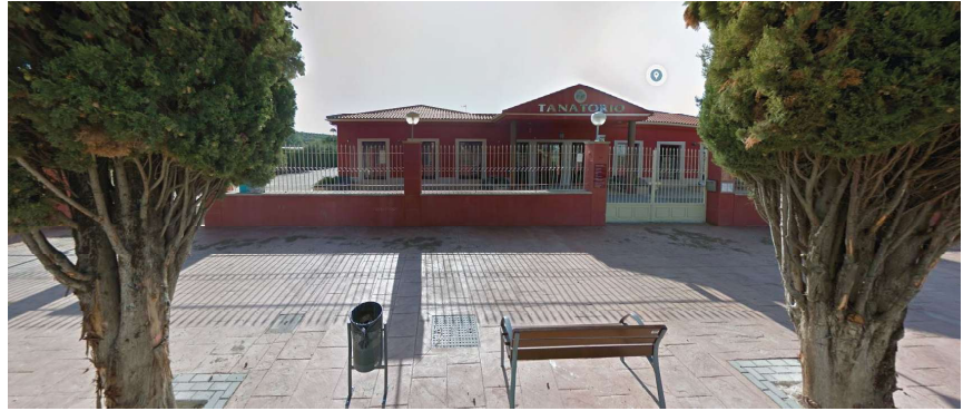
Exterior Google Street View, sept. 2019
