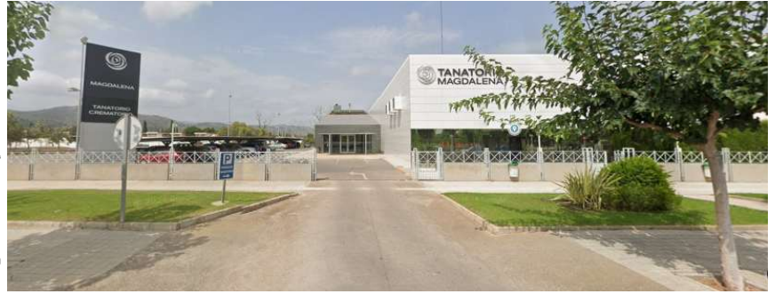
Fachada Google Street View, jul 2023
