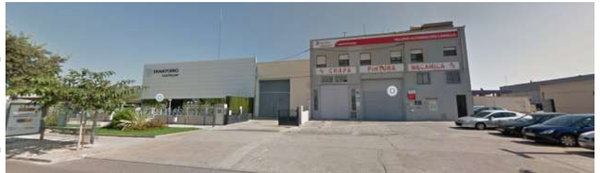
Fachada Google Street View, ago 2018
