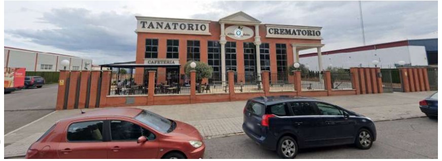
Entorno Google Street View, abr. 2022
