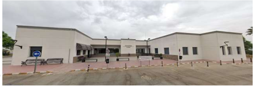
Entorno Google Street View: ago 2022
