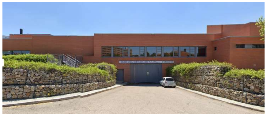
Salida f6retros. Google Street View, may. 2022
