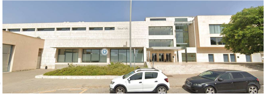
Fachada Google Street View, jul 2023
