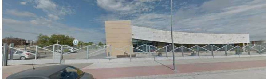
Entorno Google Street View. ago 2019
