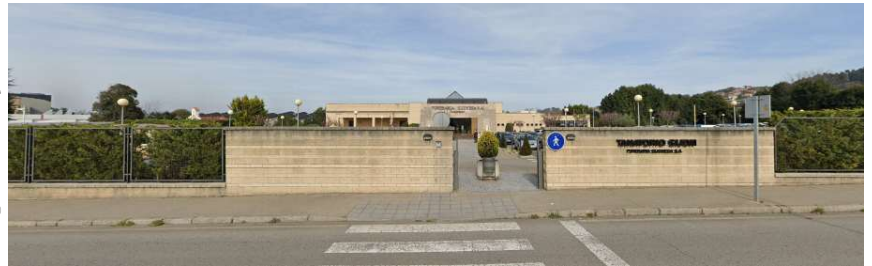
Fachada Google Street View, feb 2022
