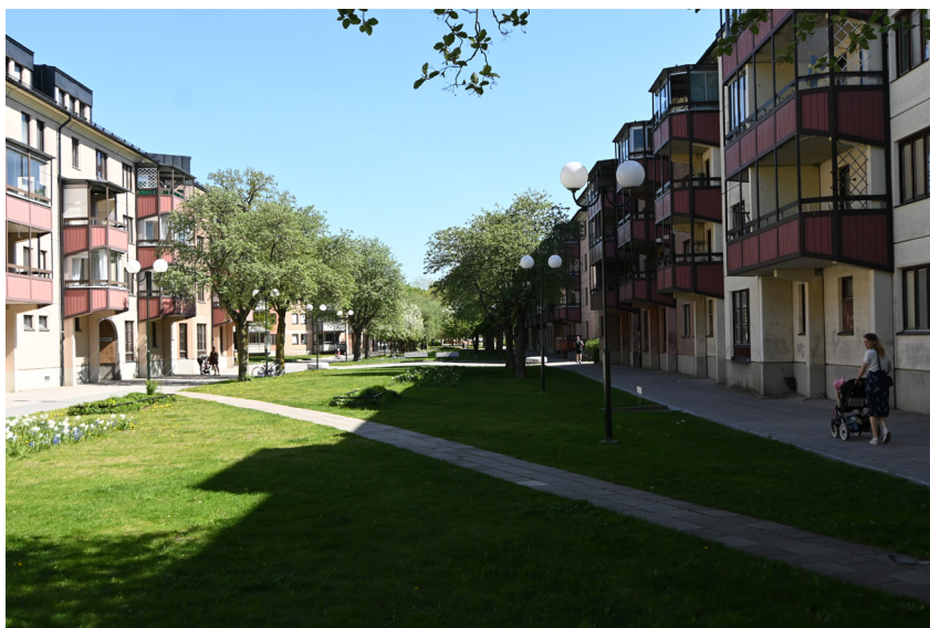
Kv. Dalen; pedestrian avenue
