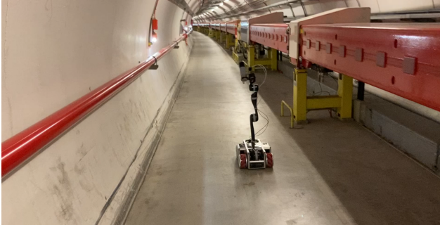
(a) Autopilot test in the SPS tunnel, maintaining a constant distance to beam components during nominal arc traversal.
