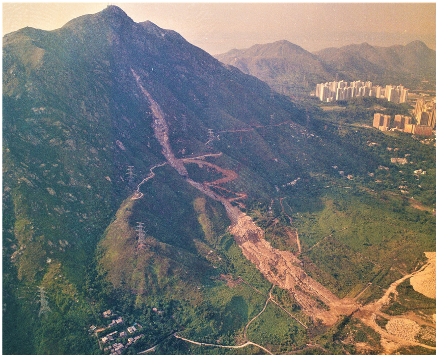
FIGURE 10 Oblique view of the debris flow (Hong Kong Geotechnical Office)
