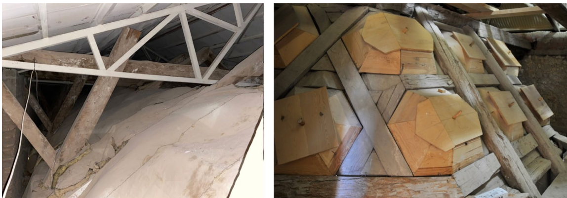
Figure 20. Comparison of the Peñaranda (left) and Pastrana (right) extrados structures. Photographs by the authors.
