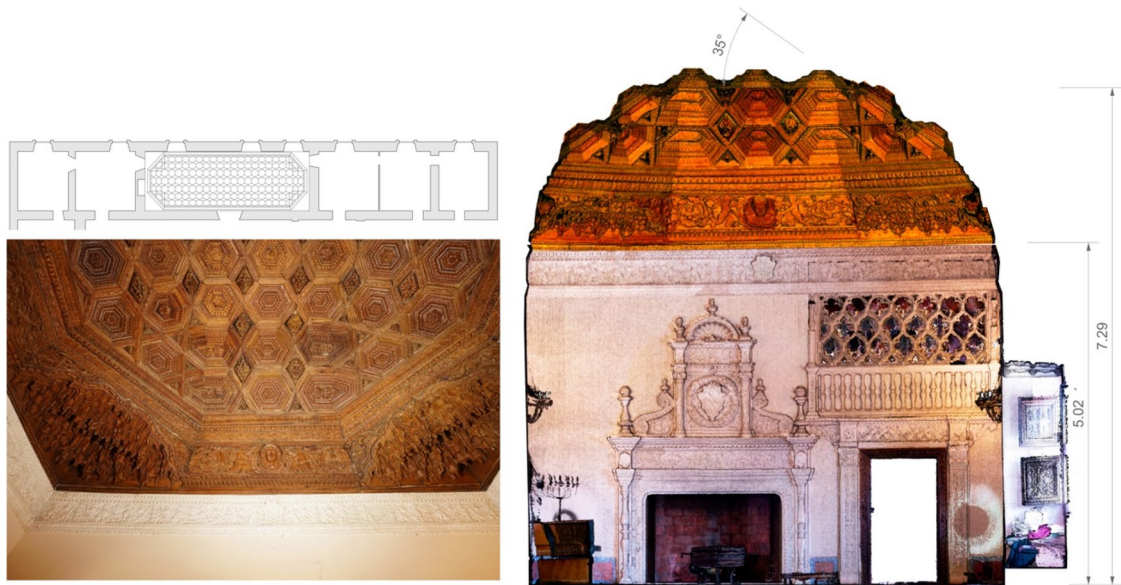
Figure 9. Ambassadors' Hall. Photograph and drawings by the authors. The ambassadors' hall is the most representative space in the building. The floor plan has a proportion of 2.76, while the section is almost a square.
