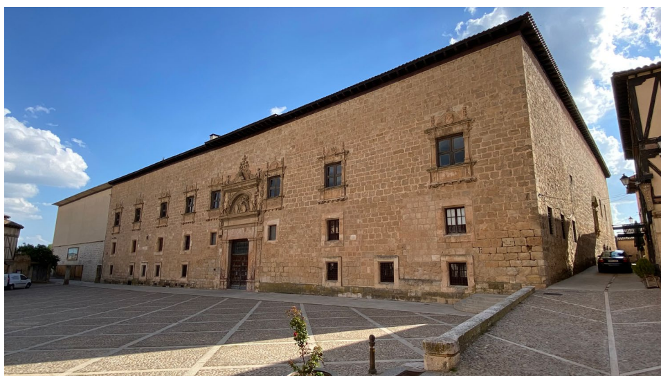
Figure 1. Palace of the Counts of Miranda in Peñaranda de Duero, Burgos. Façade opening onto the Plaza Mayor. Photograph by the authors. The raised front above the windows on the upper floor stands out. This windowless strip corresponds to the great height of the wooden ceilings.
