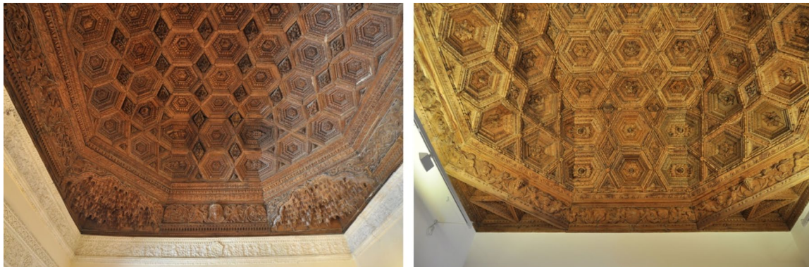
Figure 19. Comparison of the coffered ceilings of Peñaranda (left) and Pastrana (right). Photographs by the authors.
