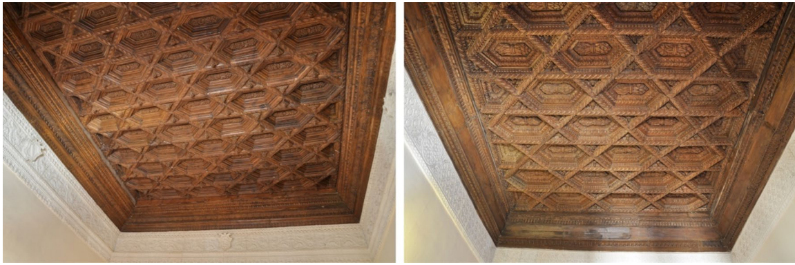
Figure 14. Antechamber and library room panelling. Photographs by the authors.
