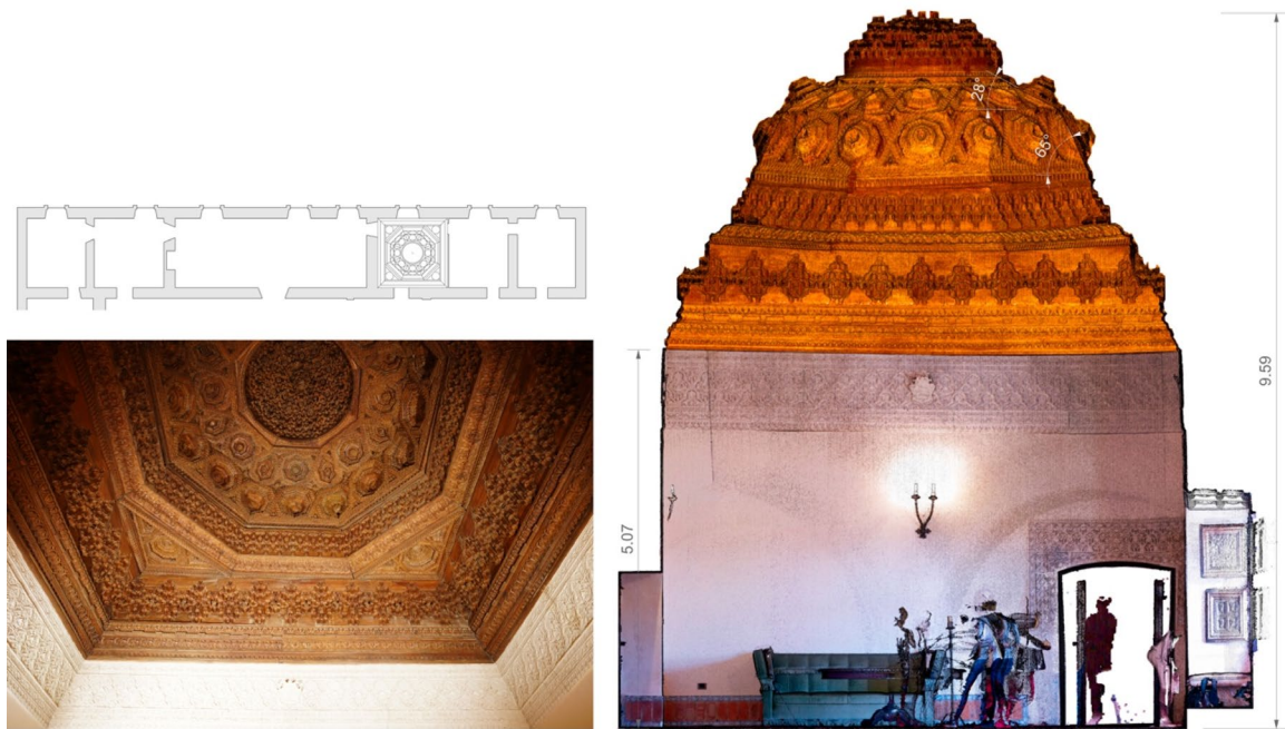
Figure 11. Hall of the muqarnas. Photograph, plan and section by the authors. This ceiling shows a delicate balance between the friezes and the muqarnas dome and the panels formed by polygons.
