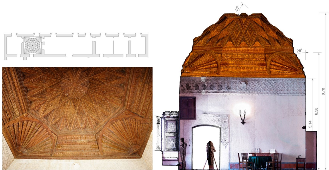
Figure 6. Shell Room. Photograph and drawings by the authors. This is a square room with an octagonal ceiling over four shell-shaped pendentives. The section is raised sharply by the 40-degree slope of the panels that form the pyramid trunk of the roof.
