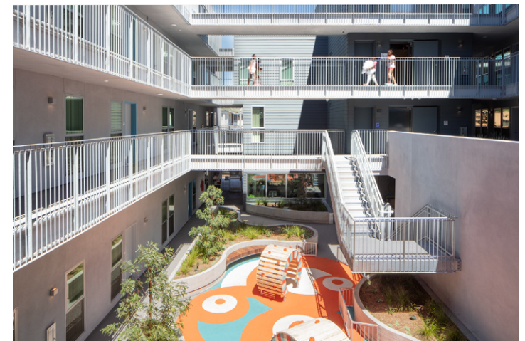
[AL] Brunson terrace, Brooks + Scarpa.
