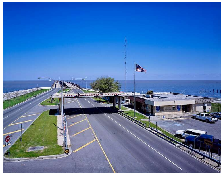
Figure 3. South Lake Pontchartrain Causeway Toll Plaza, Metairie. Source: Historic American Engineering Survey photo via Library of Congress website at https://www.loc.gov/resource/hhh.la0640.photos/?sp=2&st=image (accessed on 17 August 2024).
