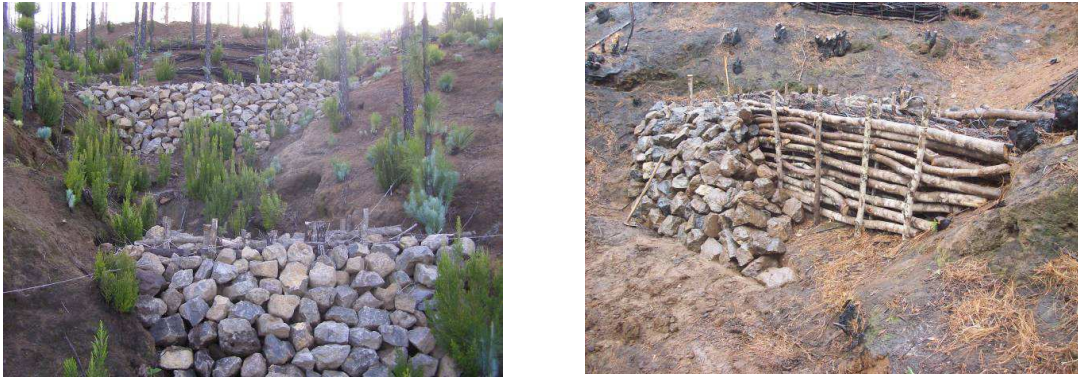
Fig. 8. Pictures of the mixed check dams evolution, effects and main elements of the design. (Photographs taken by Guillermo Tardío)
